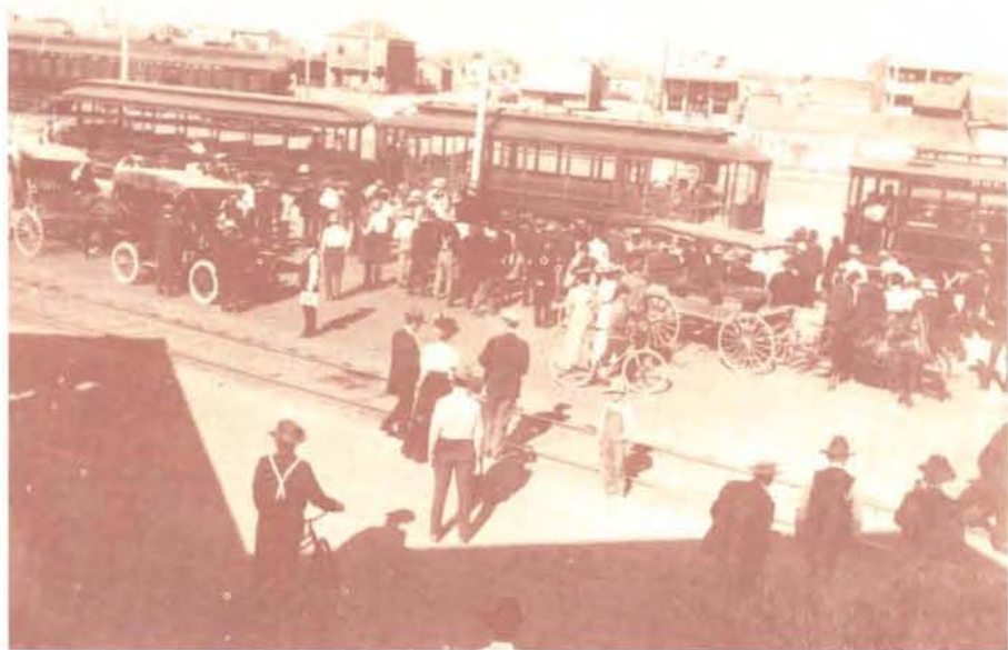
Fig. 9: Train time at the El Paso and Southwestern R.R. Station shows three types of equipment: California style car (center) hauling open trailer car (left), while passengers board a conventional (three end window) trolley at right. Photo dates from about 1916. (Photo courtesy Bisbee Mining and Historical Museum, Brophy Collection)
