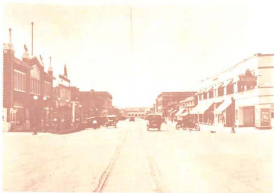
Fig. 10: The Douglas Traction and Light Company (1912-1925) was headquartered in the false fronted building (second from left) located on Tenth Street. Note streetcar track (and badly rutted pavement around it) and trolley wire in this ca. 1920 photo. Streetcar system's days are numbered as suspension of service in 1920 resulted from increased automobile ownership, declining ridership and rising maintenance costs. (Photo from Roy Manley Collection)
