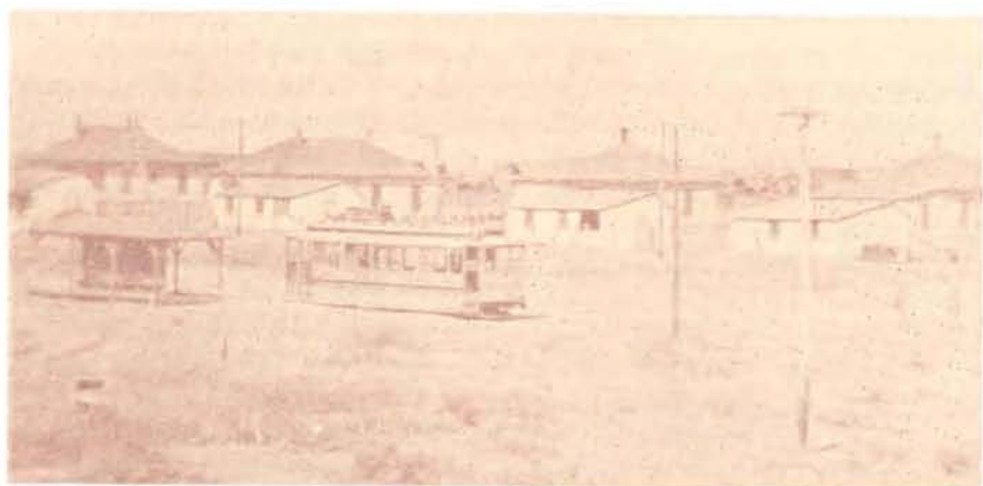
Fig. 11: A rare photograph of what appears to be San Diego car number 89 at the C & A Smelter Station, circa 1918. Both San Diego cars retained their former numbers (and paint jobs). Station is described by the old-timers in the text. Note the (mining) company town style houses and desolate look of this area. (Photo from Roy Manley Collection)
