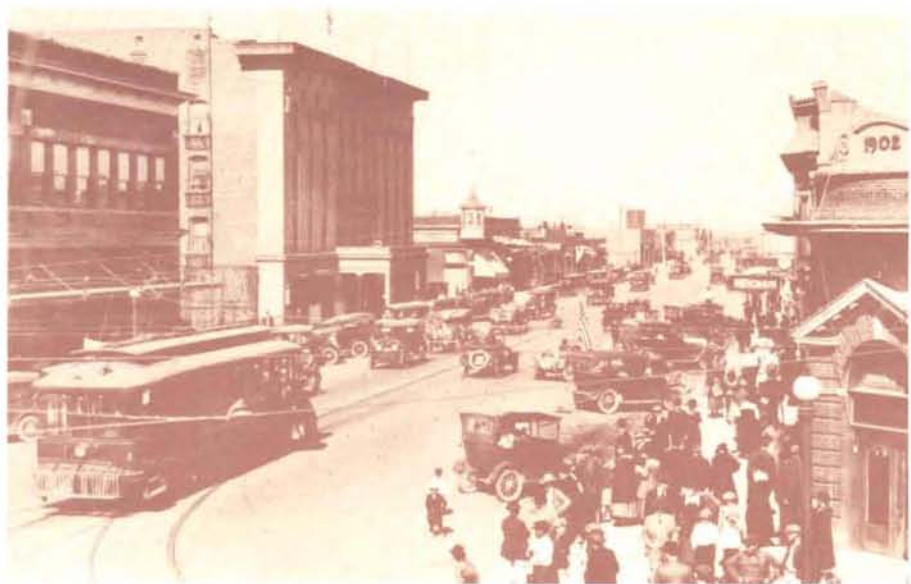
Fig. 5: California style Douglas streetcar number 1 rumbles north (away from camera) on G Avenue during the teens. Car's architecture (refer to text) and eclipse safety fender imparted a "Southern California" look to the Douglas streetscape at this time. (Photo courtesy Bisbee Mining and Historical Museum, The Cowbelles' Collection)
