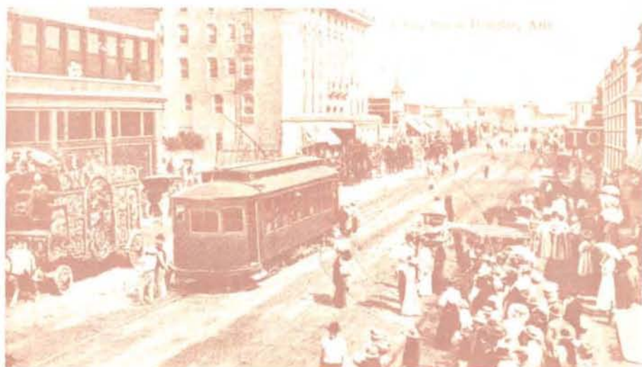
Fig. 8: A busy day (indeed) in Douglas — for the circus has come to town — finds a dark green streetcar in front of the old Gadsden Hotel and PD Mercantile buildings, running north (away from camera) on G Avenue. Note trackage leading toward right (east) on Tenth Street. Except for occasional passing sidings, all Douglas streetcar lines were single track. (Photo courtesy University of Arizona Special Collections, Tucson)
